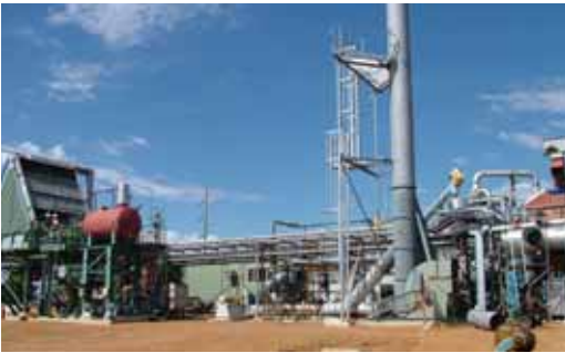
This trial plant near Narrogin in the Western Australian wheatbelt is testing the integrated production of energy, eucalyptus oil and activated carbon using biomass from purpose-grown mallees.
