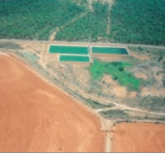
Tailings dams at Weipa, Queensland
