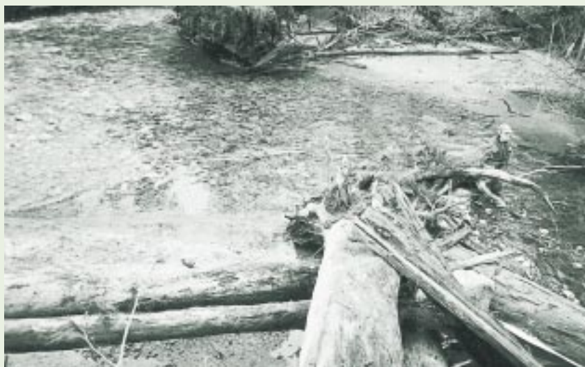
Photo 2: Log jam placed at bank in Lukwa Creek, BC to increase flow resistance, dissipate stream energy and reduce the likelihood of sediment wedge or nickpoint migration. Flow is from left to right.
