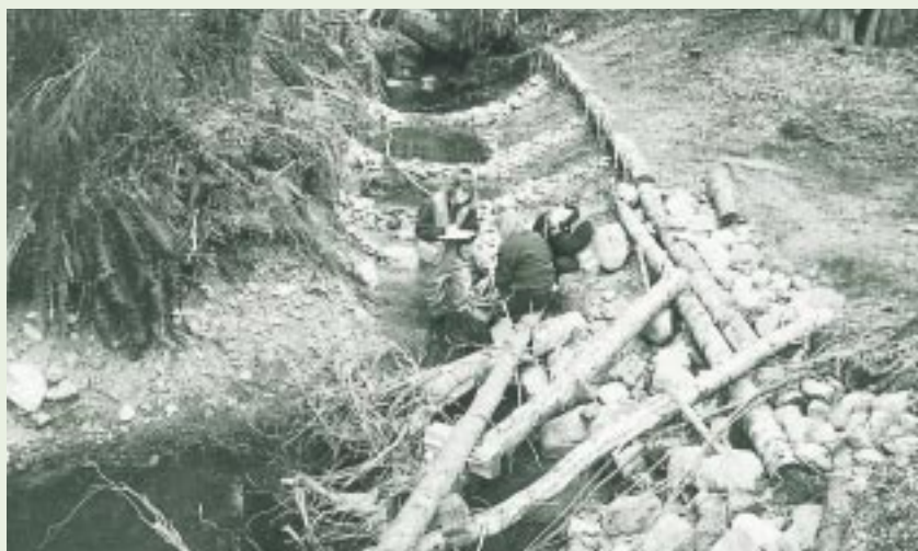
Photo 1: Wood and rock structures were placed in a tributary of the San Juan River, BC to create fish habitat and protect the banks. Flow is toward the bottom of the photo.
