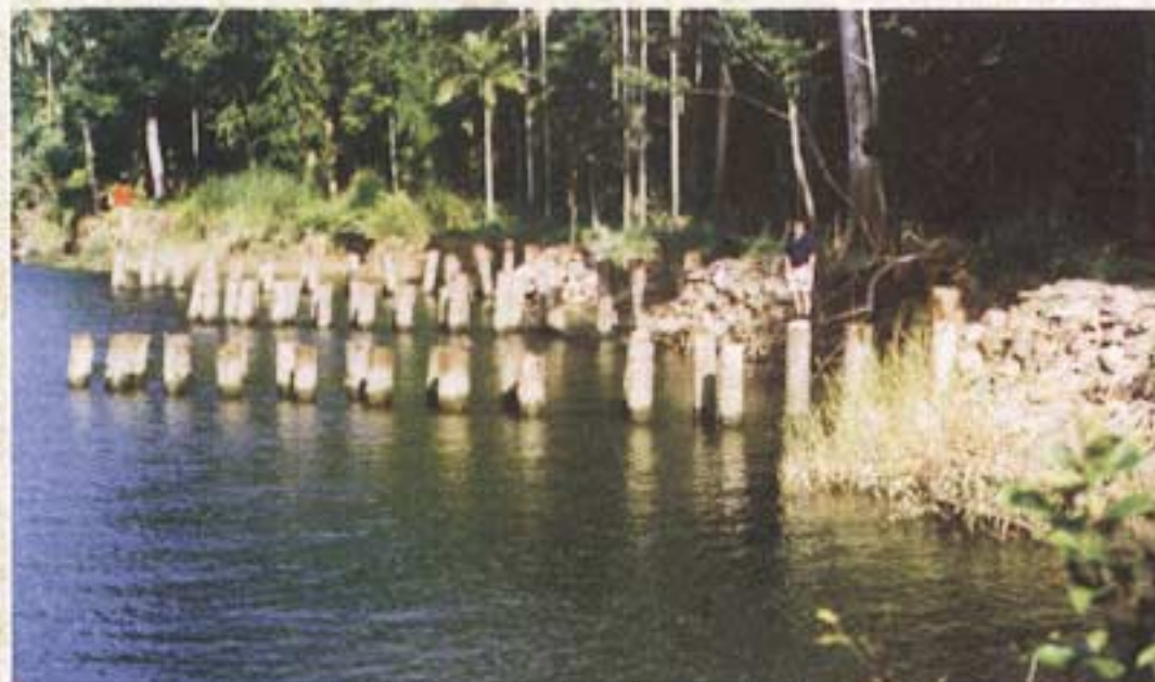
Pile groynes on the Mulgrave River
