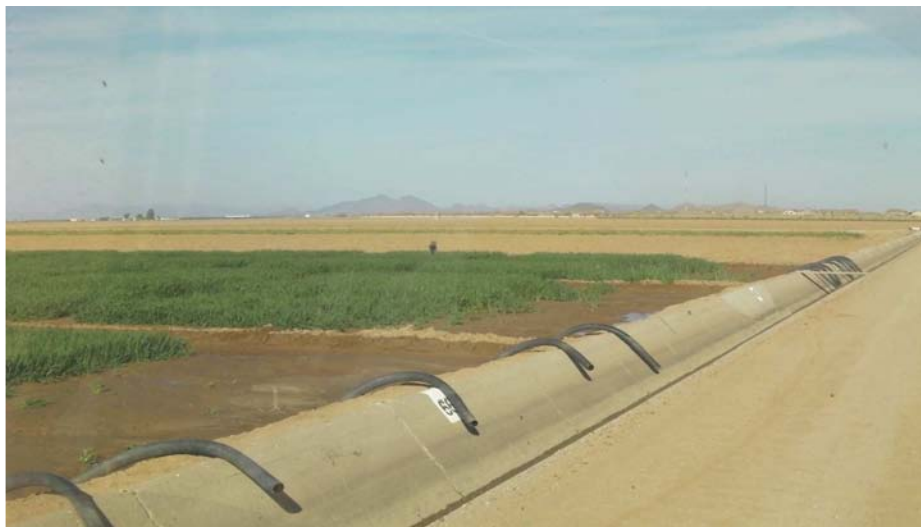
Figure 15: Furrow irrigation system from irrigation canal in the Maricopa USDA-ARS
