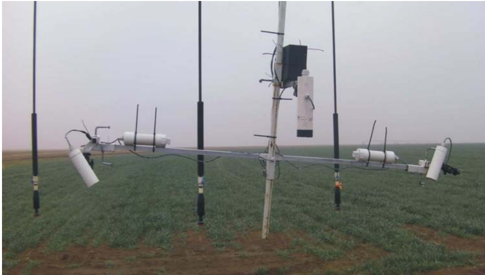
Figure 22: Three infrared thermometers on irrigation machine in Bushland, Texas
