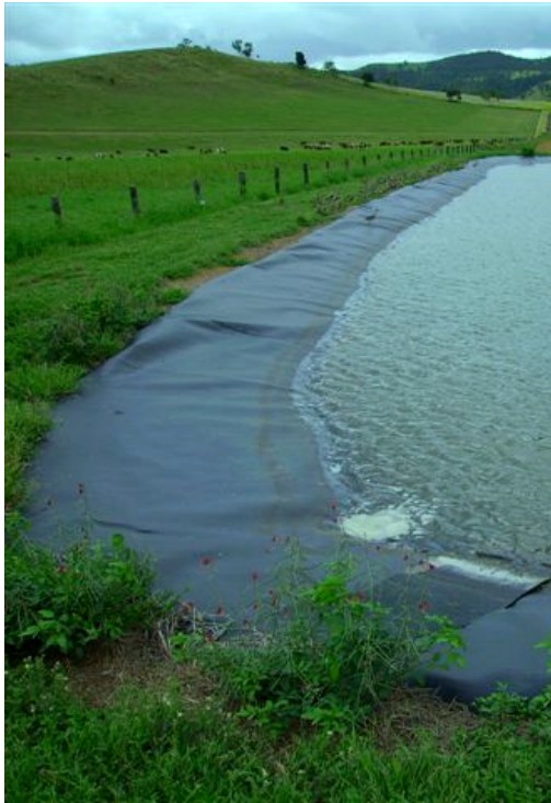
Farm Dam with Evaporation mitigation measures in place
