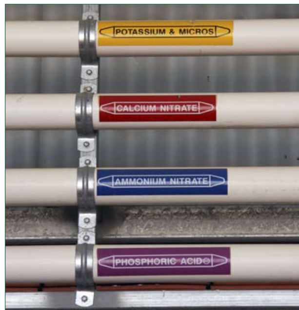
Figure 3. PVC pipes taking separate dissolved fertilisers to the injection point.
