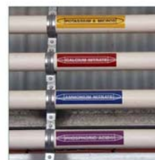
Figure 3. PVC pipes taking separate dissolved fertilisers to the pycnon point.
