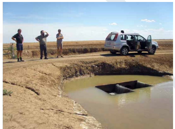
Peter deVoil and Brendan Power inspecting the irrigation infrastructure in St George at Kia-Ora with manager Hugh Mckay.
