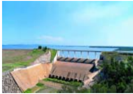
Figure 2.1 Fairbairn dam, completed 1972, capacity 1.3 \times 10^6 ML.
