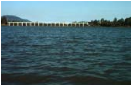
Figure 3.4 Fitzroy barrage looking downstream.
