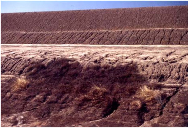
A dark patch of dead plants from arsenal used to control polymeria on a channel bank.
