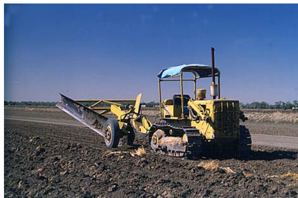
Channels are regularly re-shaped and de-silted with excavators, graders, and delvers.
