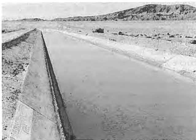
Figure 11. Sealing irrigation supply chan- nels with concrete and other suitable membranes.
