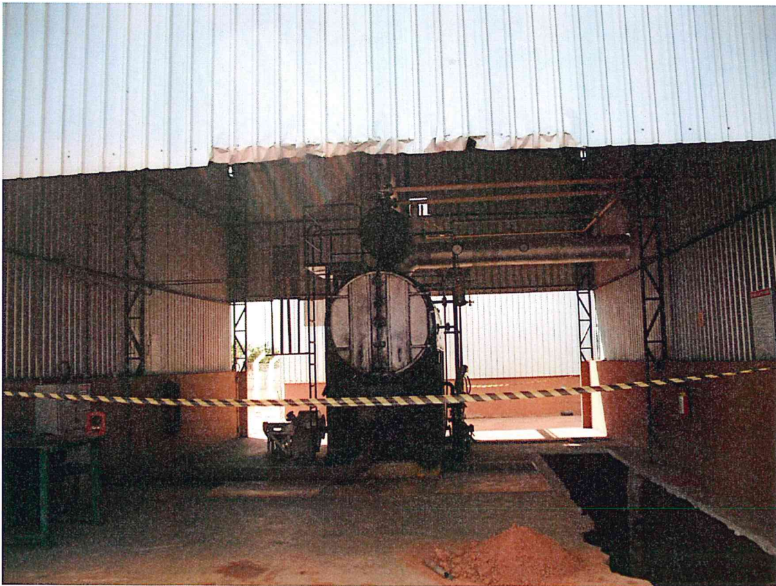
Steam boiler fuelled by cotton gin trash and timber (for adding moisture back to cotton after ginning)
