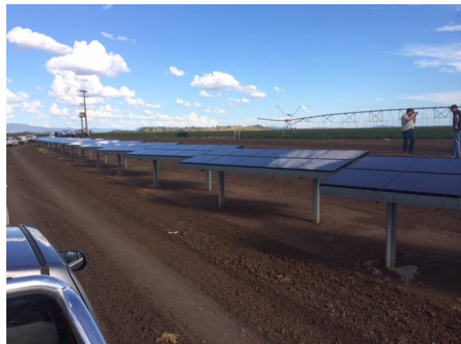
Solar panels used to power a lift pump on “Kensal Green”
