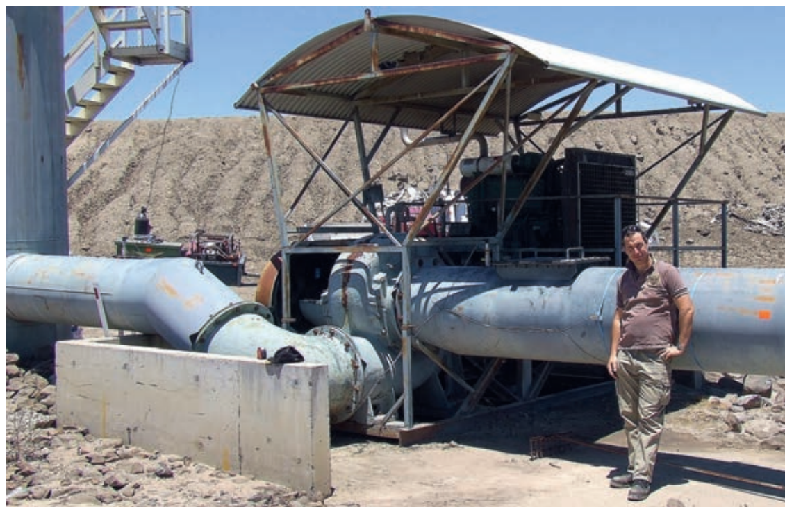
National Centre for Engineering in Agriculture's Phil Szabo installing the pump efficiency monitor at “Macintyre Downs”.
