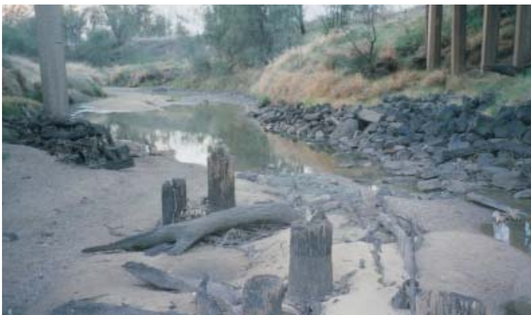
Rock riprap is being used on this part of the Condamine River to protect the toe of the bank which is gradually eroding away and threatening the bridge supports. Photo Guy Roth.
