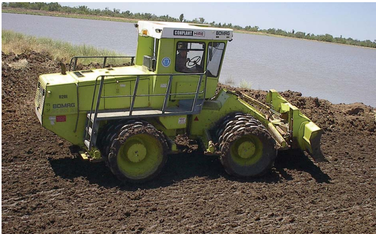
Figure 7.2. Compacting earth fill placed in an embankment breach
