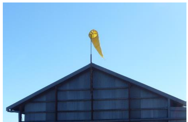
Windsocks for monitoring the wind
