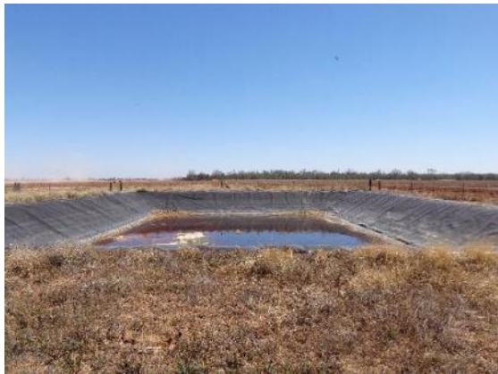
Evaporation pit lined
