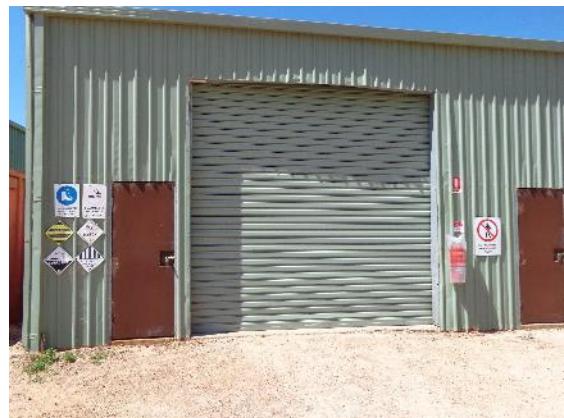
Locked chemical storage shed
