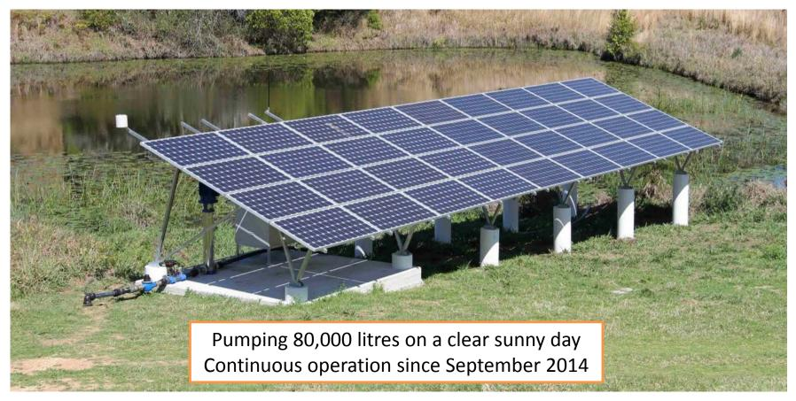
5.5kW Three Phase Pump – 60mtr Head – 600mtrs Distance – 7.2kW Solar Panel Array
