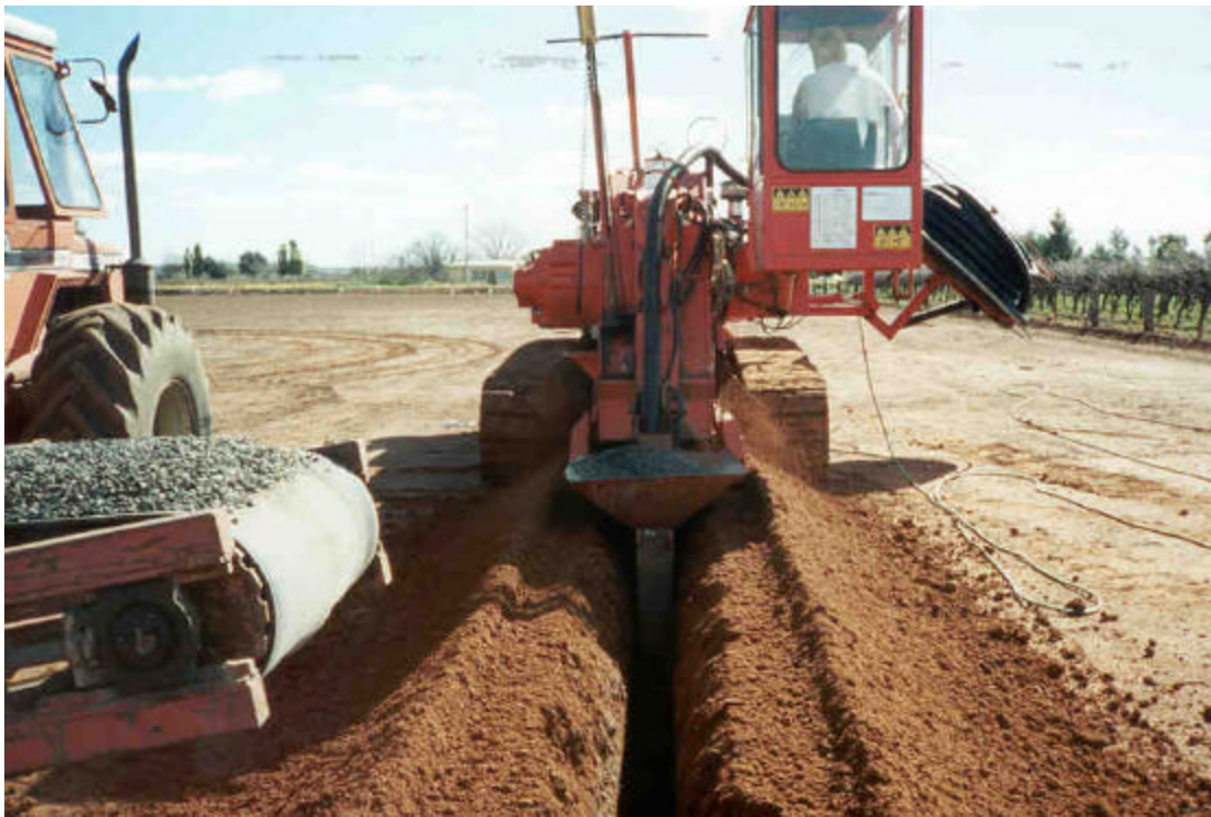
Figure 4-6. Drainage laterals being installed with a gravel envelope surrounding the drain
