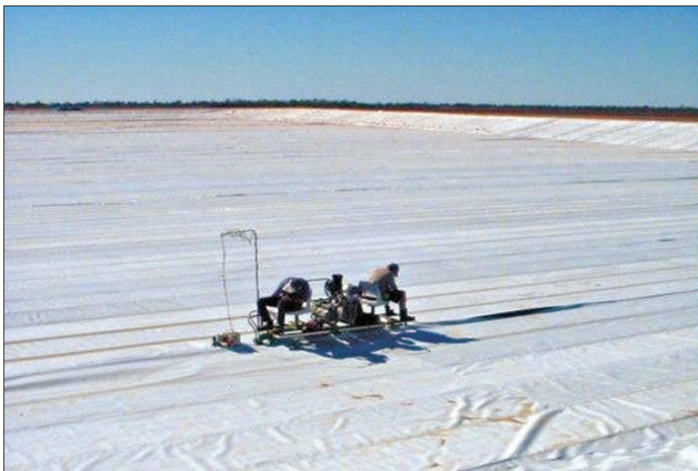
Placing of cover in progress, July 2002 (courtesy of Evaporation Control Services web site at http://www.evaporationcontrol.com.au/ )
