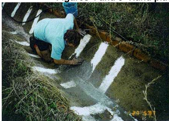
Figures 4 and 5 -Hand placement of product into joints
