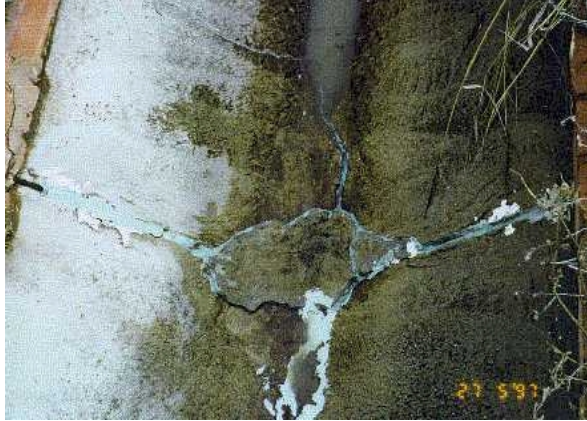
Figures 1 and 2 -Damaged channel with previously unsuccessful joint repair
