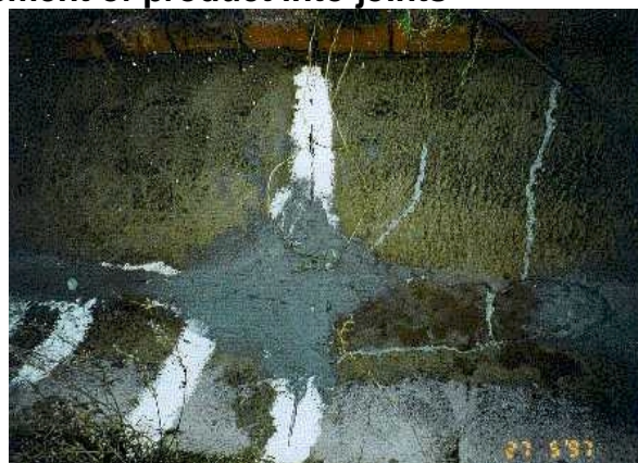
Figures 4 and 5 -Hand placement of product into joints
