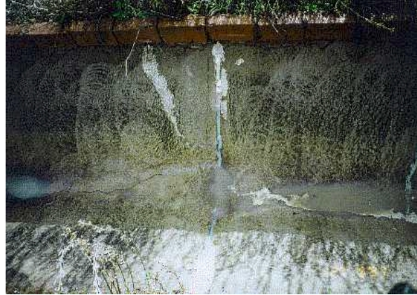
Figures 1 and 2 -Damaged channel with previously unsuccessful joint repair
