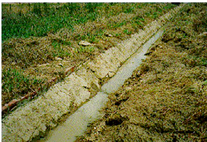
Figure 5 – Brick Topping of Concrete Channels (on left hand side of photograph)
