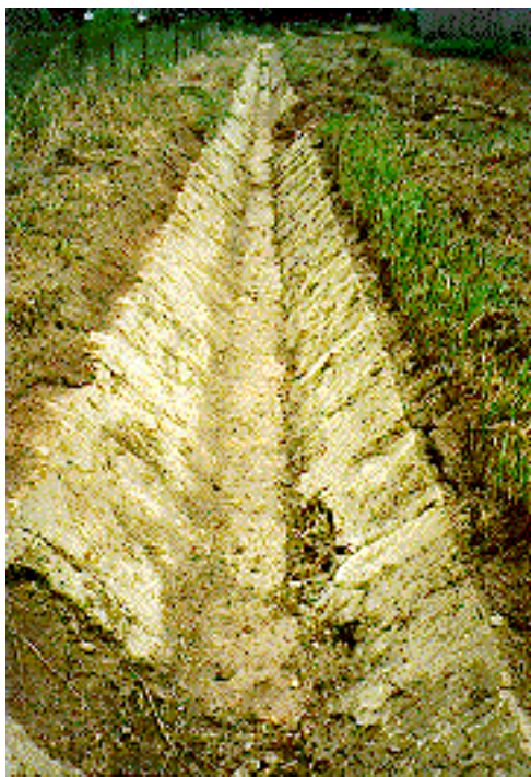
Figure 3 – Typical Small Concrete Lined Channel (note channel deterioration)
