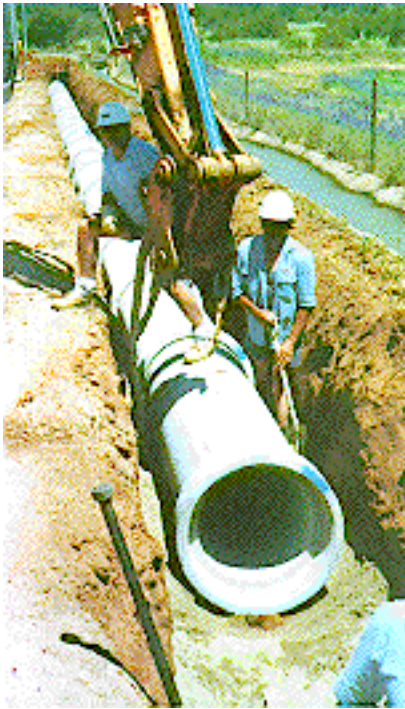
Figure 5 – 600 mm diameter concrete pipes (RRJ) being laid as part of Line D replacement
