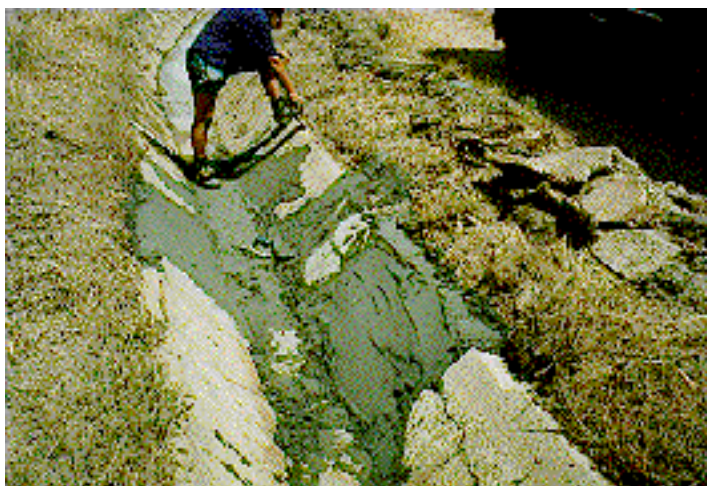
Figure 4 – Mortar Patching of Concrete Channels
