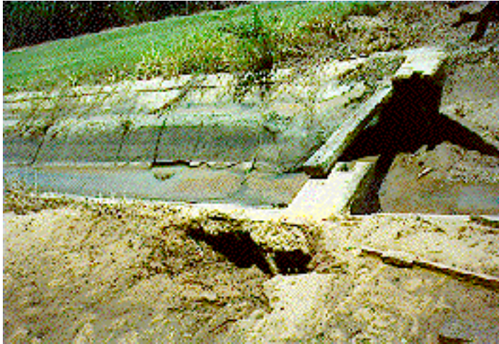
Figure 4 – Undermining of a Check Structure (resulting in bypassing of flow)
