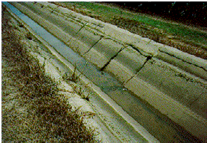
Figure 3 – Section of Concrete Lined Channel which slumped relative to adjacent section (note the detachment of capping from top of lining in right of photograph)
