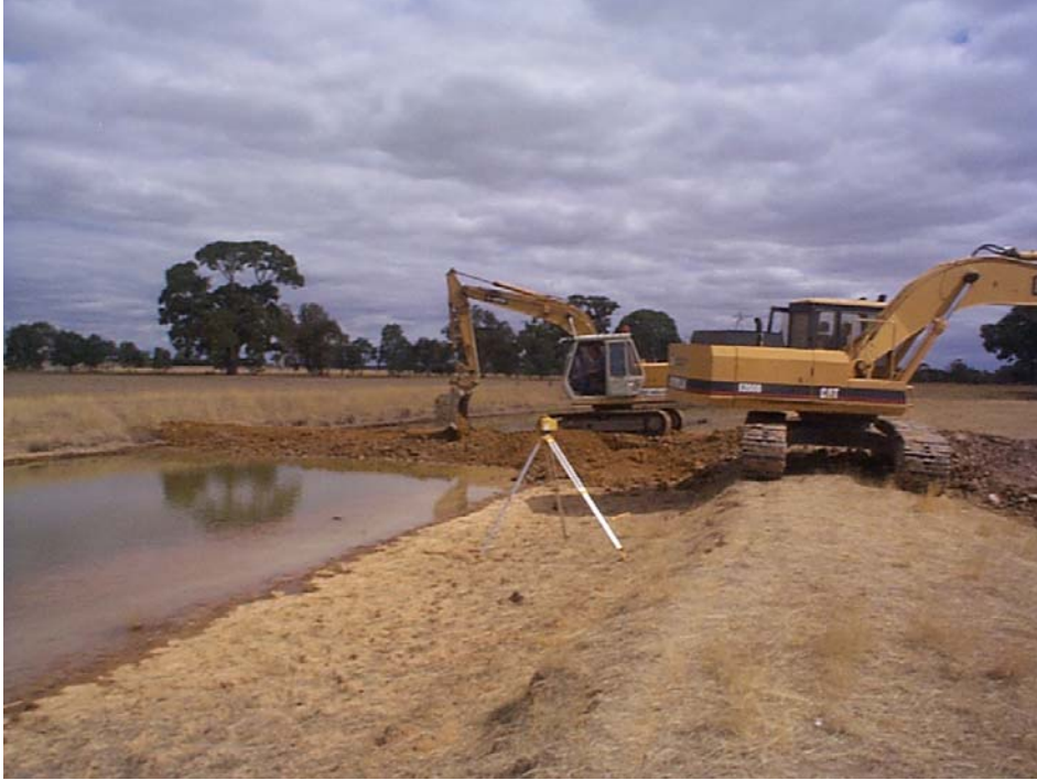
■ Figure 4-1 Pondage embankment construction (a) and installation of plastic liner (b)
