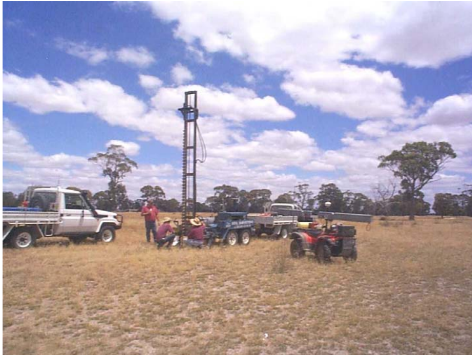
■ Figure 4-4 Trailer mounted drill rig used for soil bore drilling
