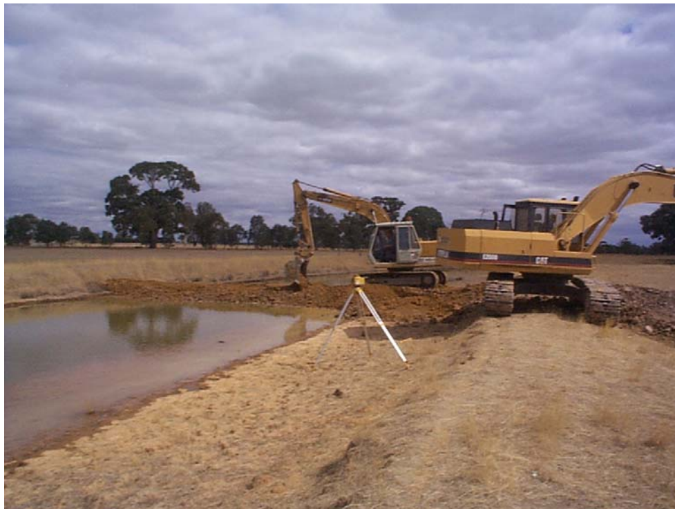
■ Figure 2-3: - Pondage test soil embankment construction
