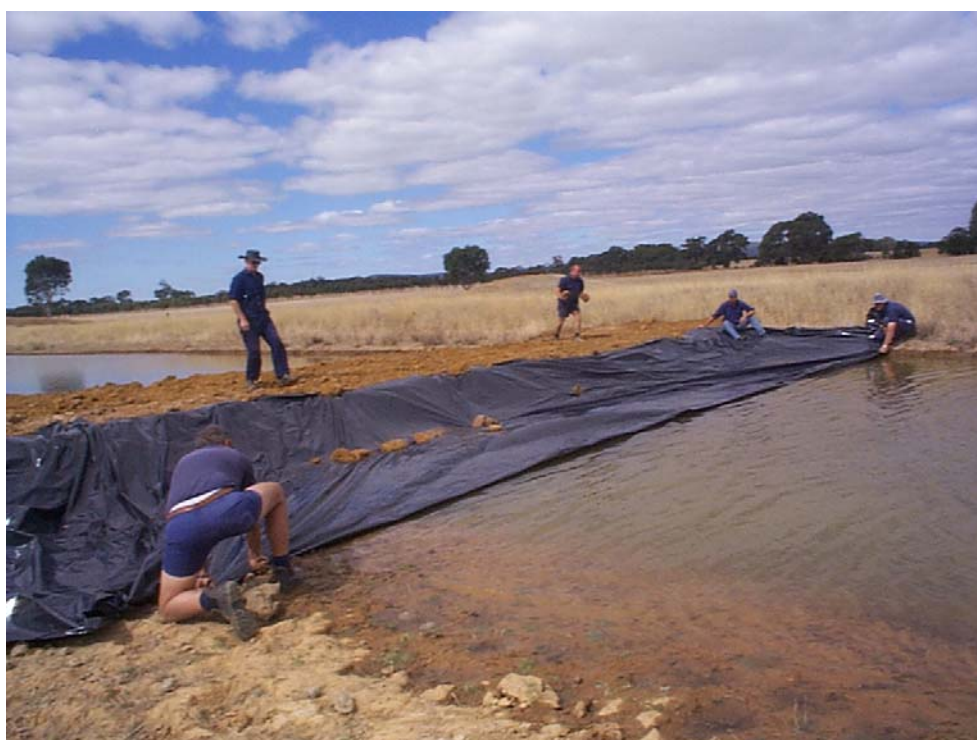
■ Figure 2-4: Pond embankment showing temporary plastic liner installation
