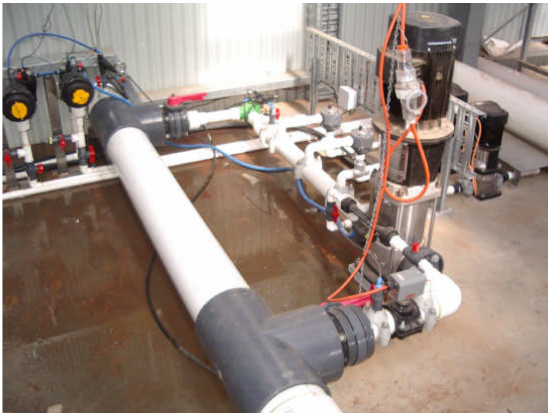
Figure 13: A centrifugal bypass fertigation system used for an Open Hydroponics program
