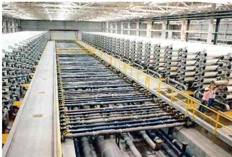
Figure 4. The process area inside the Yuma Desalting Plant, showing hundreds of pressure vessels that contain reverse osmosis membrane elements (Source: United States Bureau of Reclamation, Yuma).
