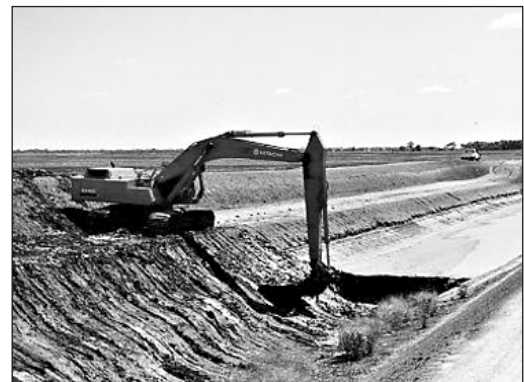
Desilting a channel.
