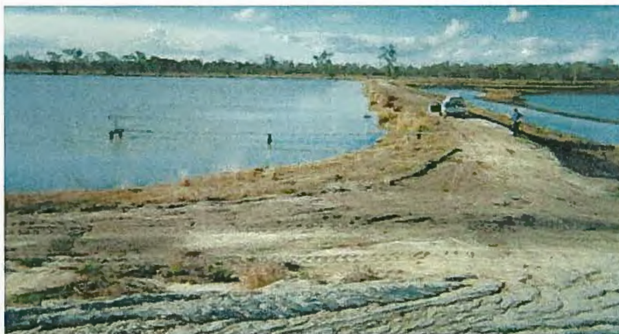
Fig 3.1 Ring-tanks are elevated earthen water storages that typically hold between 400 and 2,000 ML of water.
