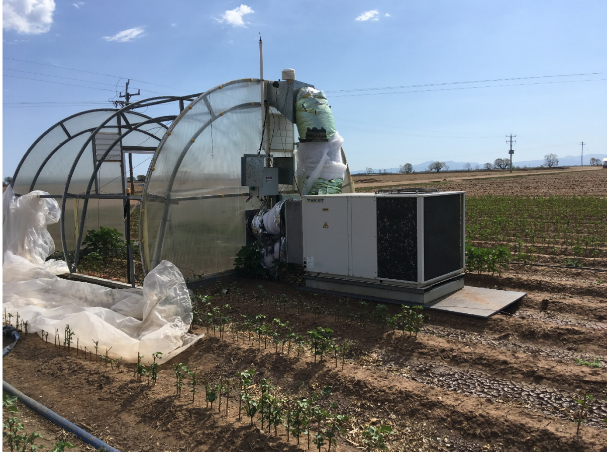
Figure 1: Storm damage to the experiment and chamber facilities during the 2018/19 season (photo taken 2/1/2019).
