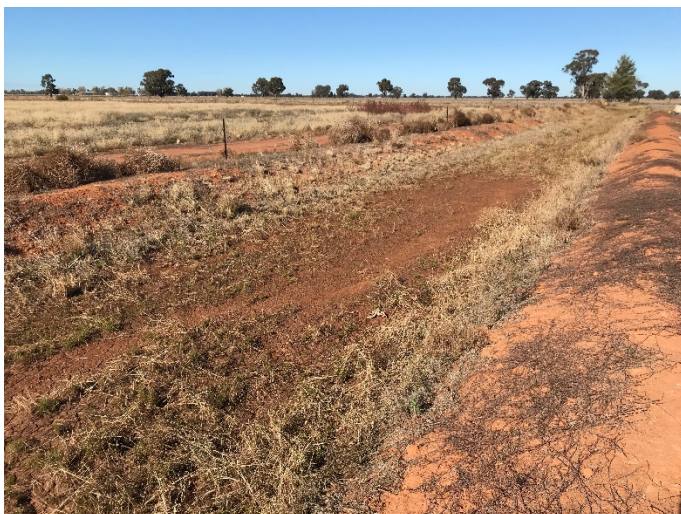
A relatively well maintained water distribution channel that could benefit from a cost-effective sprayable polymer liner to prevent weed growth and reduce seepage losses
