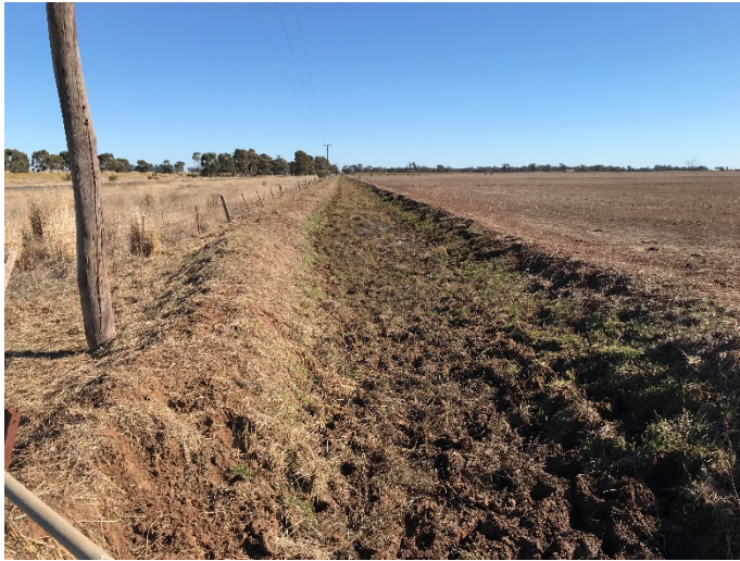
An on-farm water distribution channel damaged by animals
