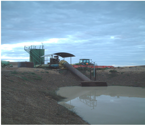
2.4b: On-farm pump site
