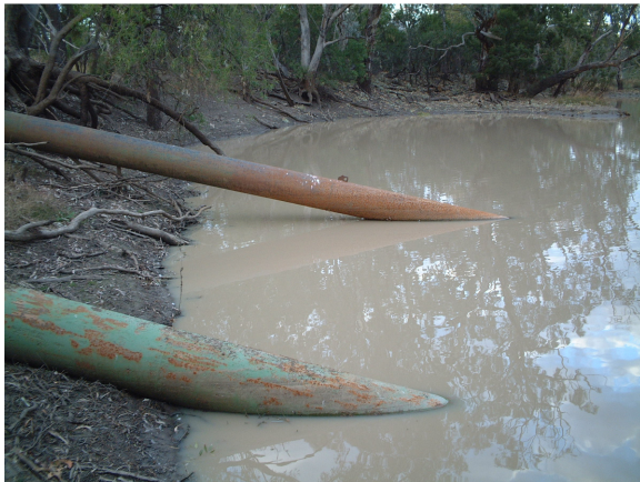
2.3b: Pipes in the river
