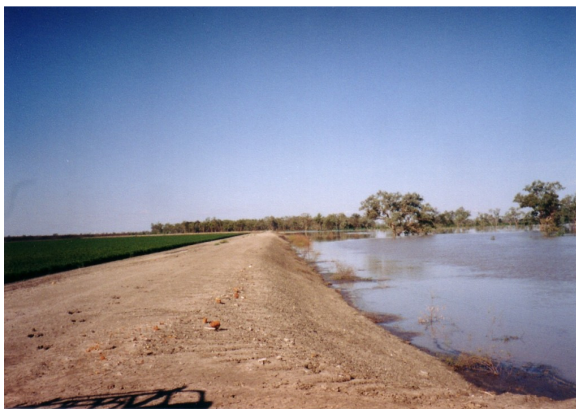
Plate 2.8: Levee bank. Photo: Susan Lutton.
