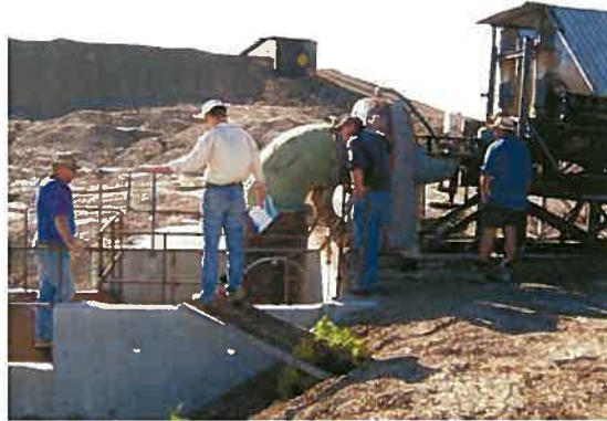
Photo 3: Walgett Pumps Efficiency Workshop
