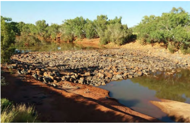
Figure 46 Recharge weir on Ashburton River (Source: Vanderzalm et al., 2018)
