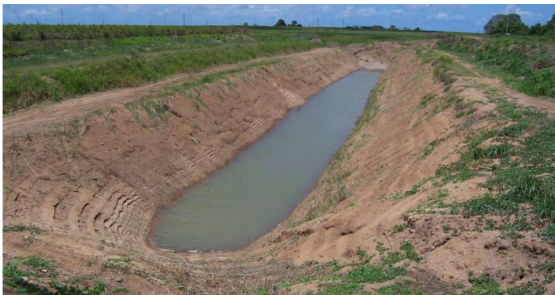
Figure 52 Infiltration basin in the Burdekin system (Source: Vanderzalm et al., 2018).
