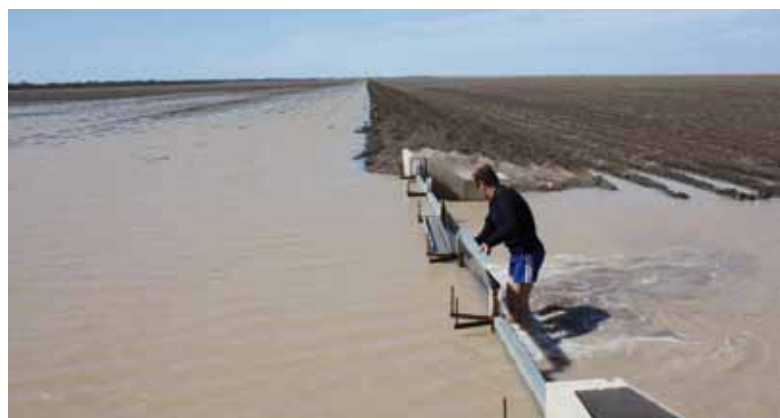
Check gates being removed between bays at a property near St George on a bankless channel system.
