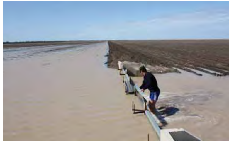
Check gates being removed between bays at a property near St George on a bankless channel system.
