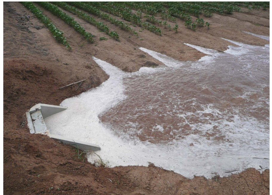
Figure 5.1.5. Bankless channel system commencing irrigation (Photo: M. Grabham)
