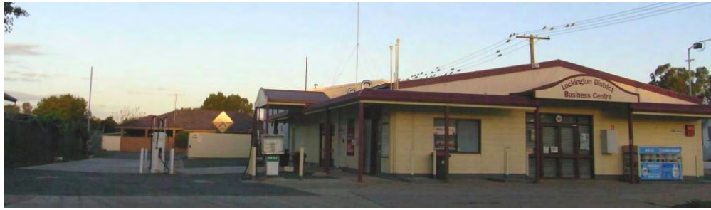
Figure 5.6: Lockington District Business Centre
