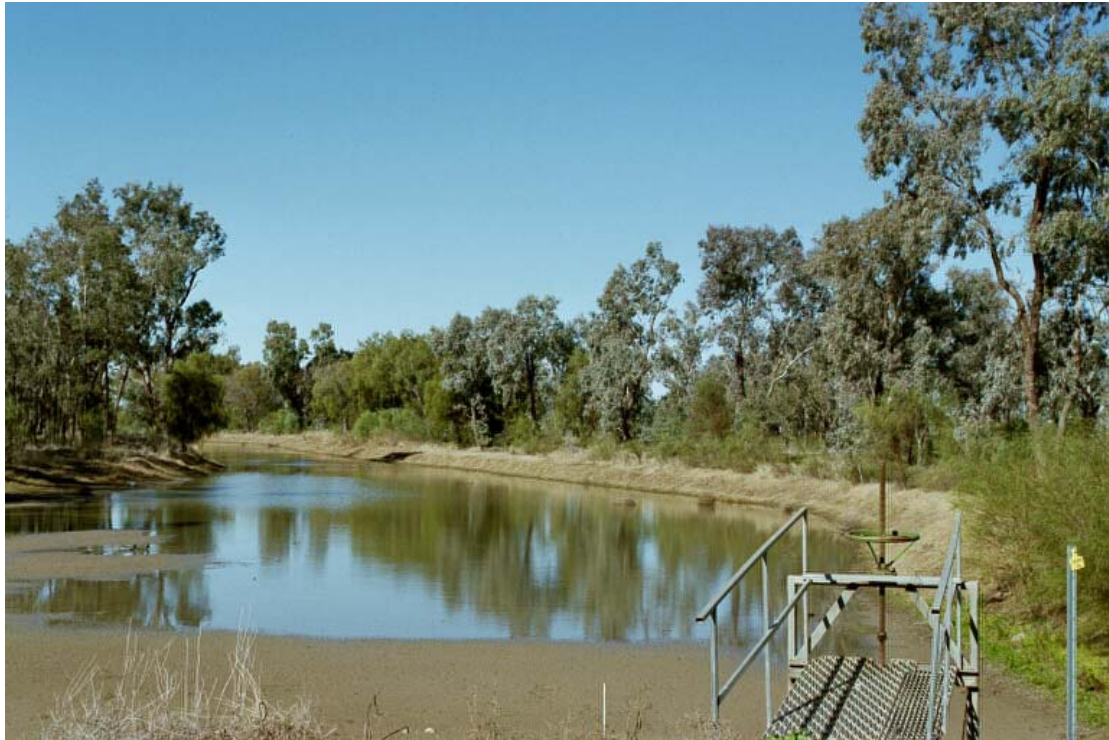
Figure 12: Irrigation main drain return established in a natural floodrunner. Naturalness of fringing vegetation retained and encouraged. Another of the most productive sites.
