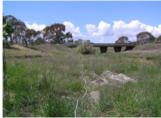
River Oak (RVC 71) on Cobrabald River (order 4) New England Tablelands (Score = 34. Poor condition)
